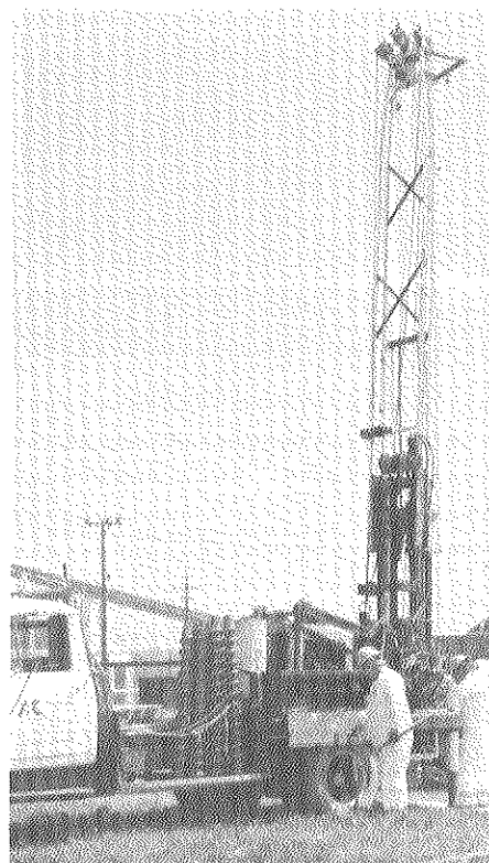
Geraghty & Miller Environmental Services and subcontractors are performing the field investigation of the RCRA Facility Investigation (RFI). Eight rigs are being used during the drilling phase of the RFI.
